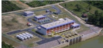
INTAKE WORKS AT SG. SEDILI BESAR
