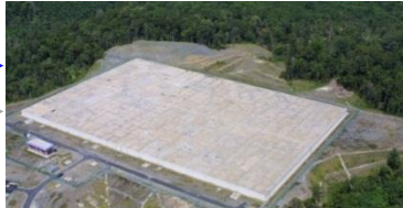
TERMINAL RESERVOIR AT BKT. PANJANG
